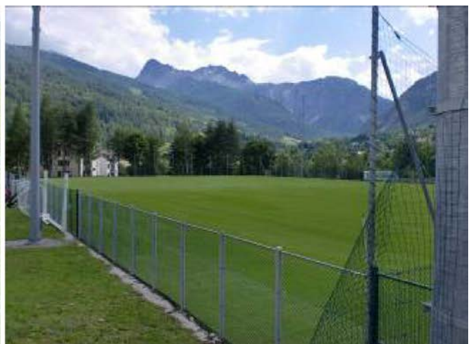
The new lay of the field with DuPont™ Typar® geosynthetic covered with the natural turf
